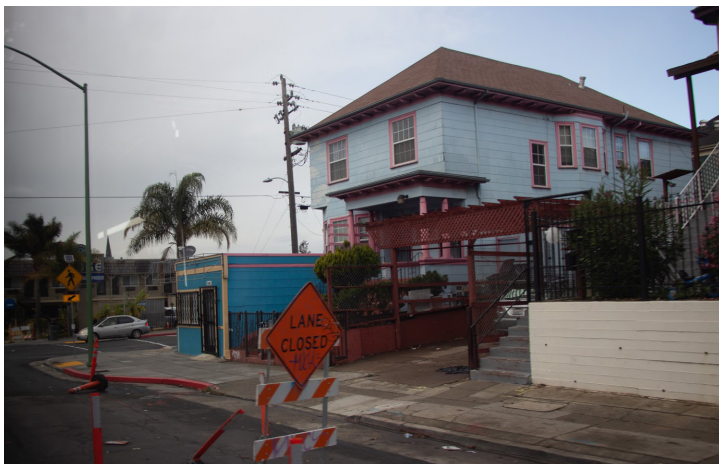
Figure 12. Current Housing Impacted by Construction on International & 15th Avenue
