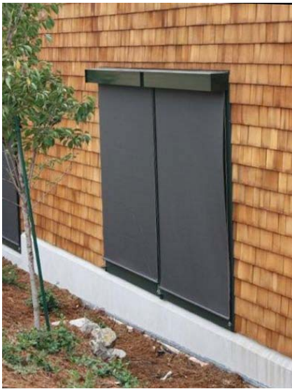
Figure 2: Automated exterior roller shades on west elevation (left) and shade detail (right)
