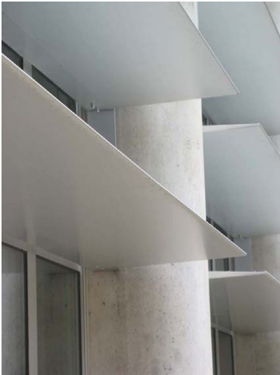
Figure 50: Detail of aluminum louvers
