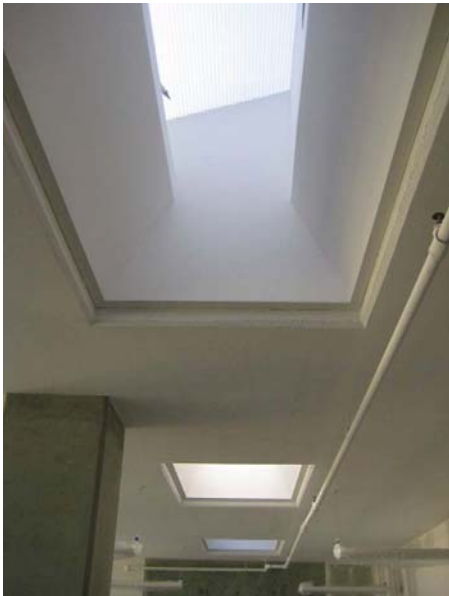
Figure 52: View of 4th floor skylights
