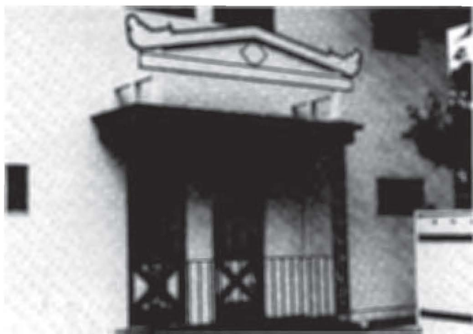
Existing building at Westminster Memorial Park, redesigned for use by the Orange County Vietnamese community.
