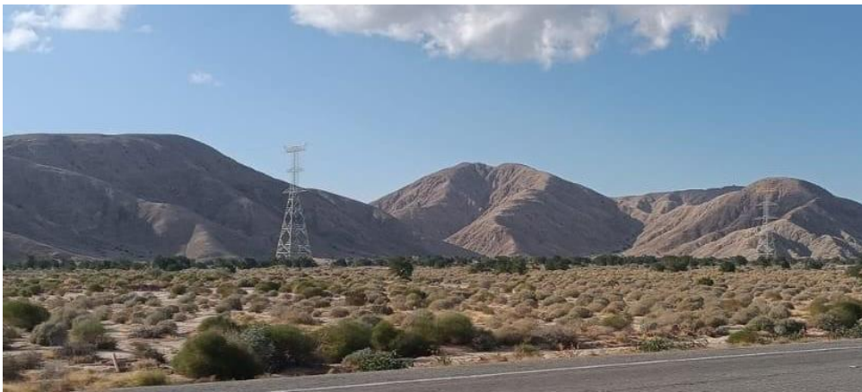
Figure 3.2 CFE new electric towers in Cucapáh collective lands. Photography. 2023 (Márquez, F.)
