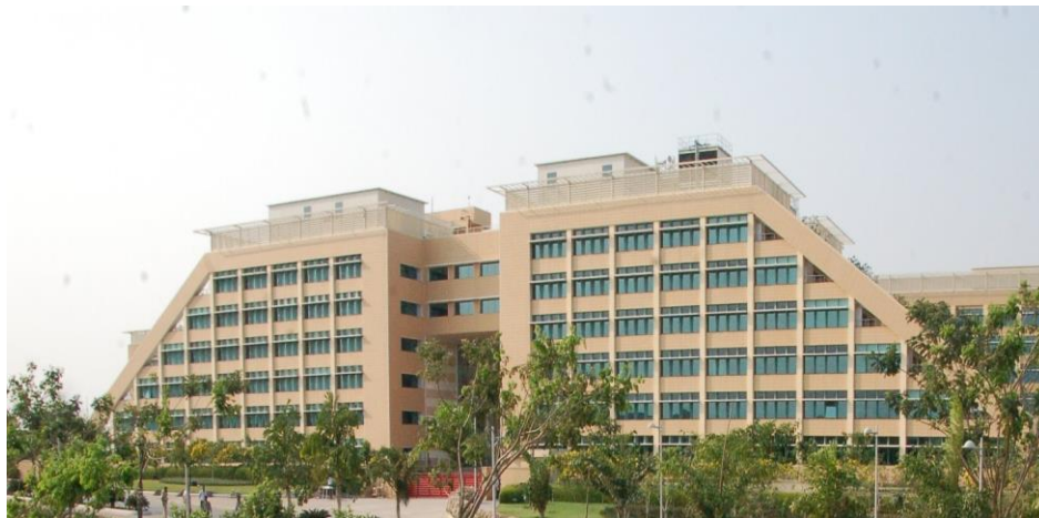
Figure 1. The Pocharam SEZ Campus, Hyderabad. One half has a VAV cooling system and the other half has a radiant slab cooling system, which consistently uses 1/3 less energy than the VAV system (Sastry and Rumsey 2014).
