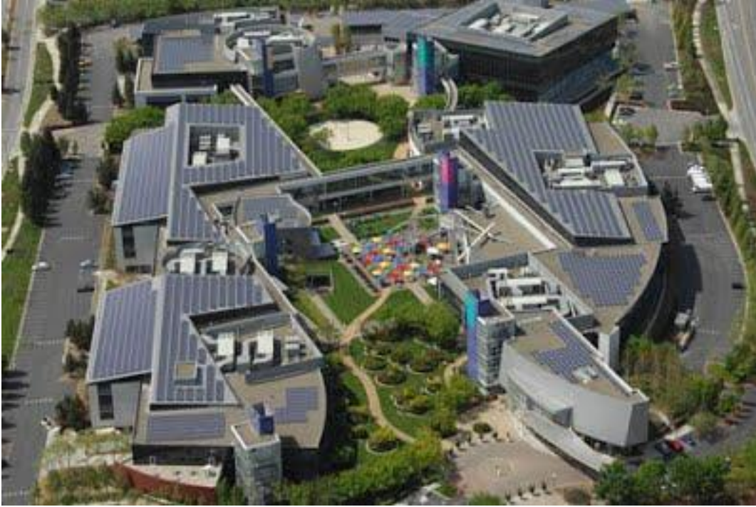
Figure 2. Aerial view of the "Googleplex" Google's Headquarters in Mountain View, CA, showing the photovoltaic panels on the roofs
