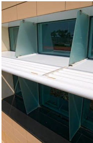
Figure 4. Window detail, showing overhang / light shelf and translucent side fins.
