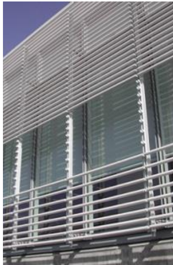
Figure 1. Example of high performance façade used on the New York Times HQ tower in NYC. Consists of “layered” design solutions, A) inside-to-outside and B) floor-to-ceiling. A) consists of 1) External fixed ceramic rods for shading for solar control and daylight diffusion; 2) High performance insulating glass unit with spectrally selective low-E coating, argon gas fill and low-iron glass, including some fritted sections for glare control; 3) Interior automated, motorized roller shade with shade material selected to balance daylight admission and glare control. B) consists of 1) plenum and upper glazing zone for glare control and light diffusion; 2) central unobstructed vision area; 3) lower partially shaded zone that admits daylight to bounce off the unoccupied floor area adjacent to window. ( Lee et al, 2005)
