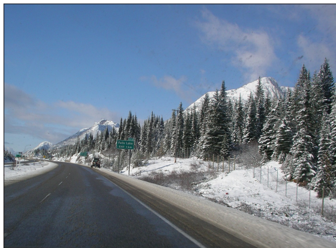
Figure 10. Wildlife exclusion fencing on the Coquihalla Highway.
