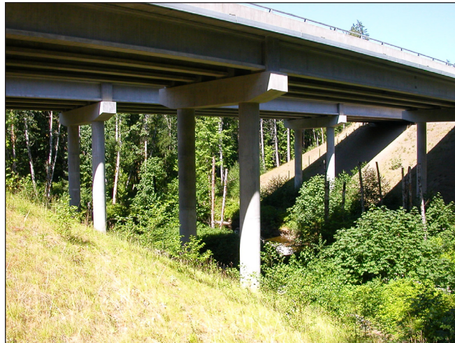
Figure 7. Multi-species wildlife underpass on the Vancouver Island Highway (1999).
