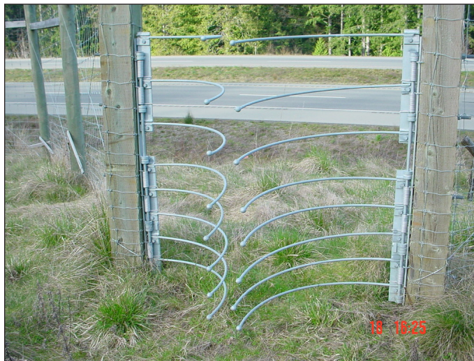
Figure 2. One-way gate designed for moose and deer.
