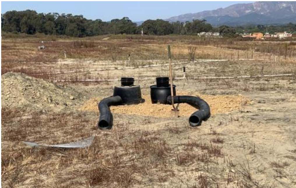
Figure 48. Breeding artificial burrows designed by David Johnson. These include a halved 55-gallon drum laid over hardware cloth, 10' long 6" tunnels, curved for darkness. Cut and glued into the tops are 3.5-gal buckets with the bottoms cut out. A second, soil filled bucket is placed inside these as a plug to insulate from noise and temperature. The “plug” bucket can be removed and allows for access and banding of owlets.
