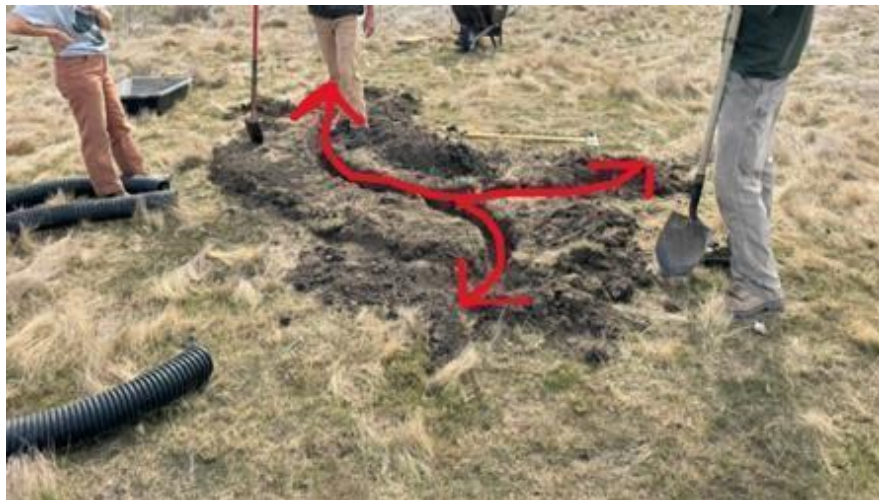
Figure 46. Winter burrow design being installed at Hollister Ranch. This burrow is made of 4" corrugated pipe, with a "Y" at one end, allowing the owls to choose their preferred aspect, and escape from raptors from three different directions without the need for pivoting abruptly in the air to enter. These are easily plunged periodically for maintenance. Designs with two or four entrances can also be constructed. 6" designs should be installed for comparison. 6" is preferred for room to maneuver inside but is more accessible to skunks, opossums, and where they occur, badgers. Burrow reducers or rebar driven off-center inside the entrance can prevent that.
