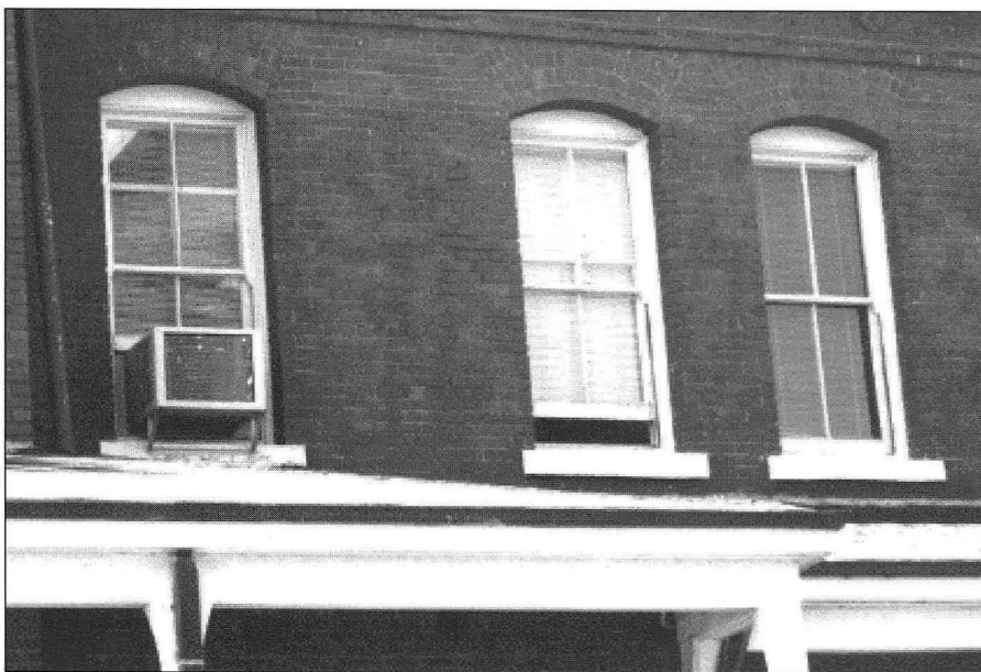
The open window in the center provides free ventilation and cooling. Ironically, the unnecessary air conditioner on the left prevents similar use of that window and damages the building's historical integrity.
