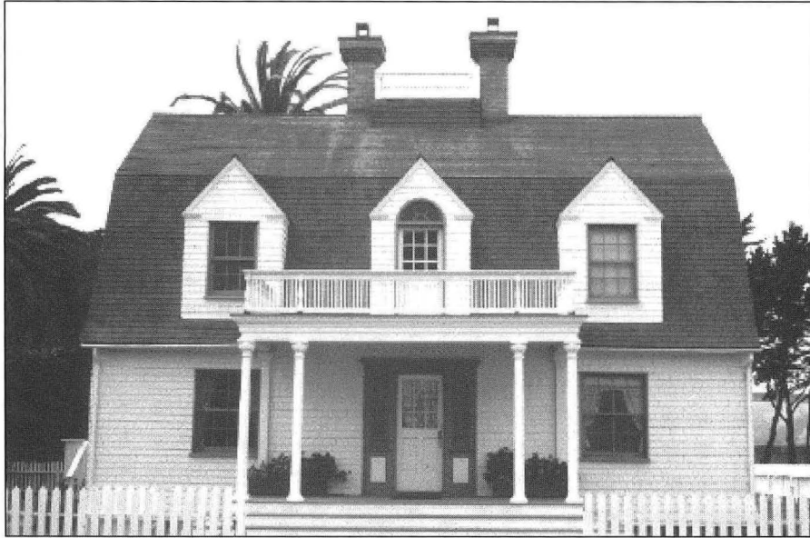
Historical architectural features, such as overhangs and porches, provide structural shading and windbreaks.
