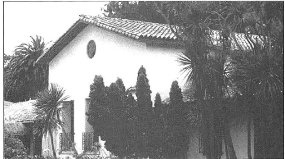
Air flows under the barrel tiles on this roof, removing the sun's heat before it enters the occupied areas of the building.
