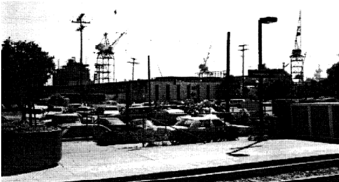
Figure 3: View from Harborside Station, looking west toward National Steel and Shipbuilding
