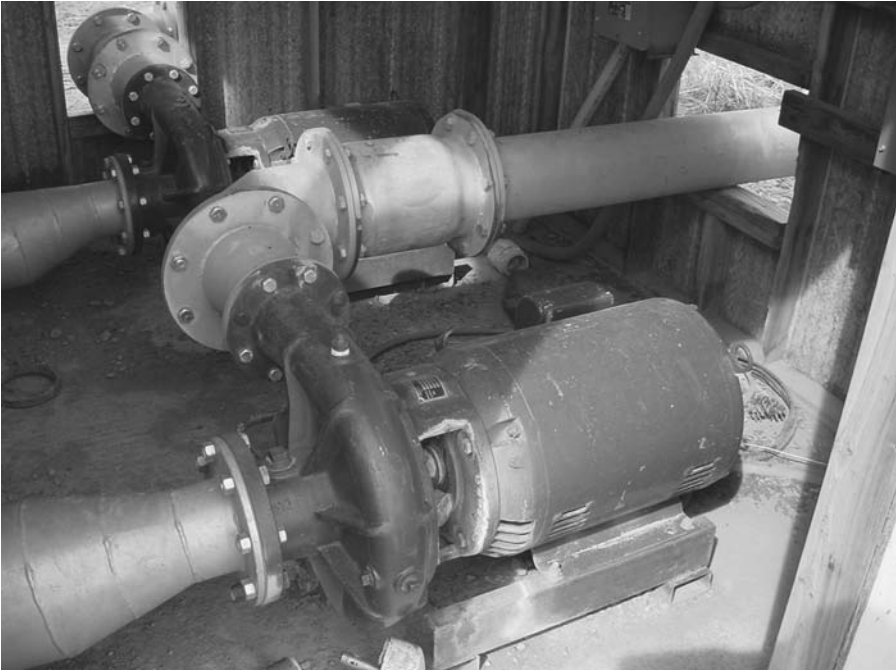
FIGURE 4. Large electric water pumps used to draw water from a nearby irrigation ditch and supply irrigation equipment. Photo by T. Acker.
