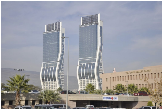
Fig. 3 200 m high Twin Folkart Towers in Bayrakli supported on a piled raft system. No earthquake-induced damage was identified or reported for such foundation systems
