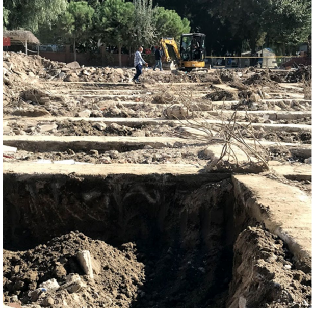
Fig. 2 Two-way combined footing system (grid spread footing foundation) of one of the heavily damaged buildings in Bayrakli, whose collapse is not foundation induced
