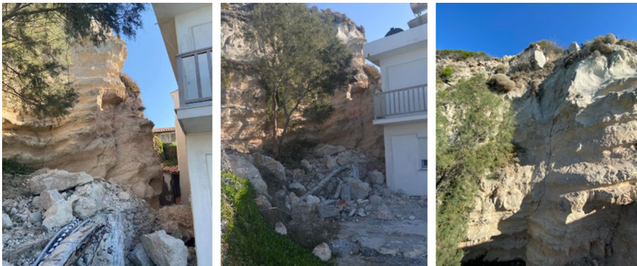
Fig. 22 Detachment of sandy marls and marly limestones recorded very close to a residential building in the Kokkari region (photos taken by the HAEE/ETAM reconnaissance team, 37°46'49.9" N, 26°53'35.0" E). Vertical open cracks are visible, clearly susceptible to detachment and toppling
