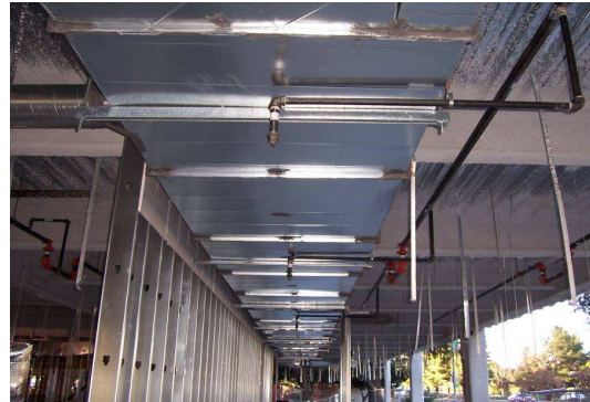
Figure 8: Priority Wall on Camino Project (Source: DPR Construction, Inc. Redwood City, CA)
