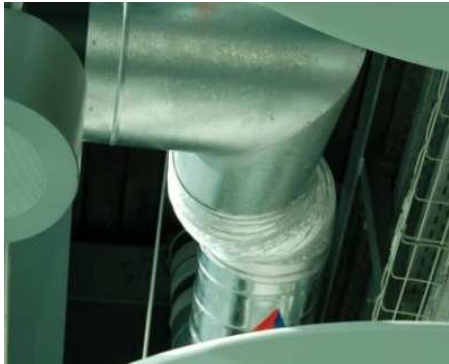
Figure 7: Flexible duct connection absorbs dimensional variation (Source: Iris D. Tommelein)
