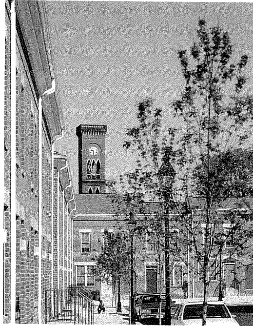
View of street edge and corner along main square, looking south. Photo: Torti Gallas/CHK
