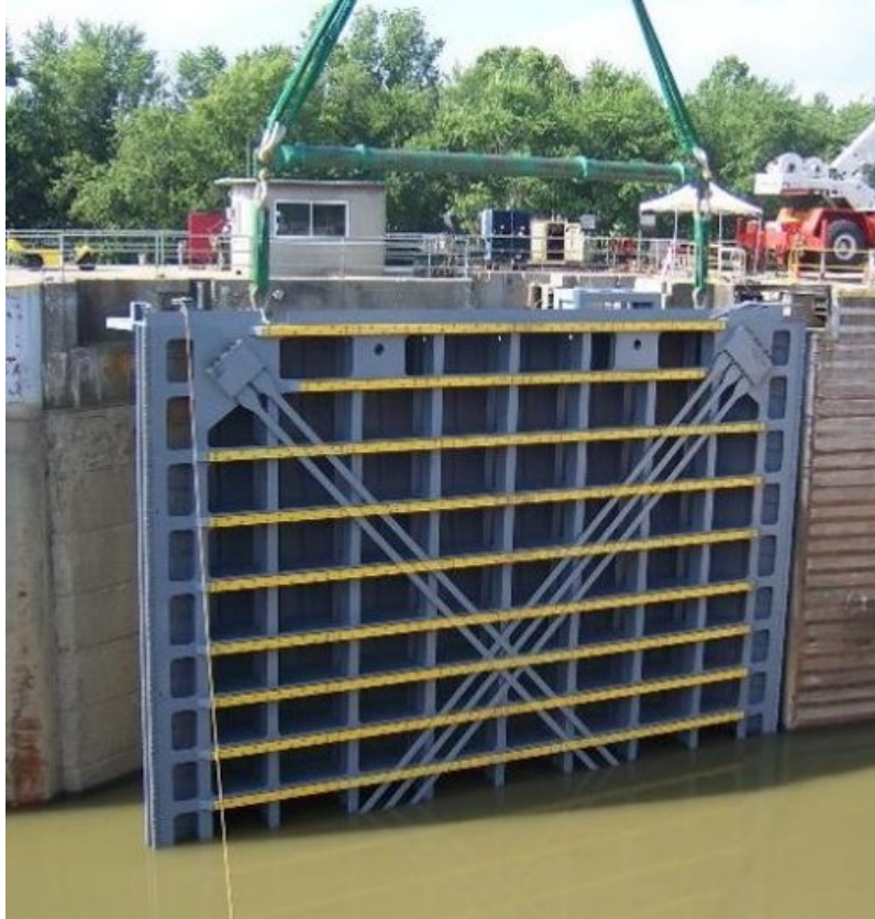
Figure 2.1. An open miter gate.
