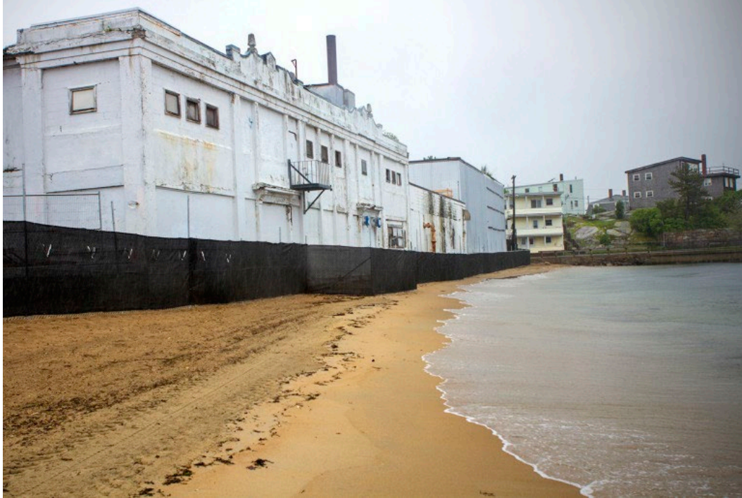
Figure 3.1 A photo of Pavilion Beach and the Birdseye facility. This was taken before its demolition and redevelopment of the property as the Beauport Hotel. Photo credit: Kuhlmann, A. (2016, June 22). Beauport Hotel opens doors to Birdseye, Frozen Food Pioneer . The Gloucester Clam. Retrieved April 9, 2022, from http://www.gloucesterclam.com/2016/06/22/beauport-hotel-opens-doors-to-birdseye-frozen-food-pioneer/ .
