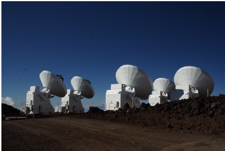
Figure 3.3 The Submillimeter Array, located at 13,400ft atop Mauna Kea. There are 8x6m dishes that are used primarily in the submillimeter bands. Credit: Katherine Alatalo
