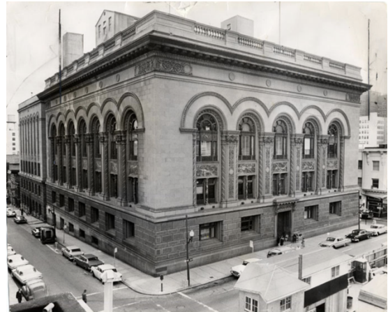
Figure 31: The rebuilt Hall of Justice and county jail of San Francisco. This site was later occupied by the Holiday Inn.
