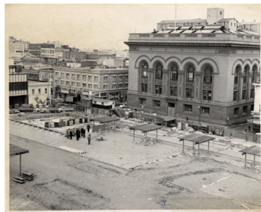
Figure 24: Royston's design in construction atop the Portsmouth Square garage.
