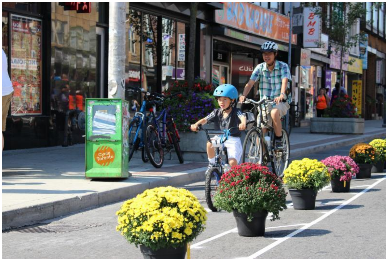
Figure 82. Class IV planter protected bike lanes, Toronto, Canada Source: Cycle Toronto (n.d.)
