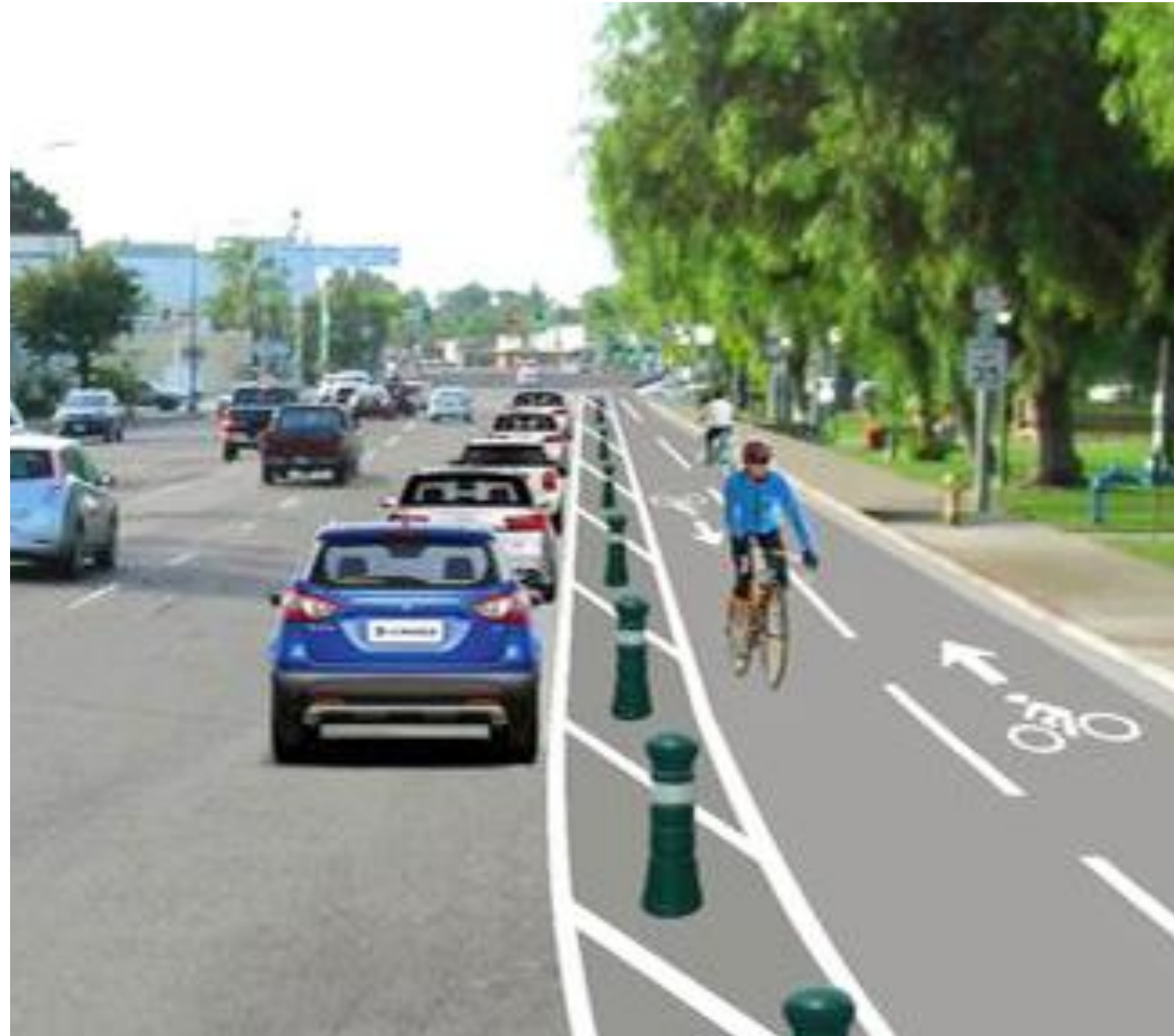
Figure 68. Class IV two-way bollard protected bike lanes Source: City of Escondido, CA (2018)
