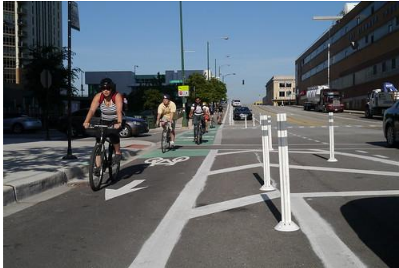
Figure 55. Class IV plastic bollard protected bike lane Source: ChicagoCompleteStreets.org (n.d.)
