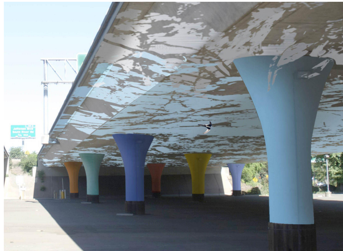
Figure 45. Underpass mural, Sacramento, CA Source: Sactown Magazine (2016)
