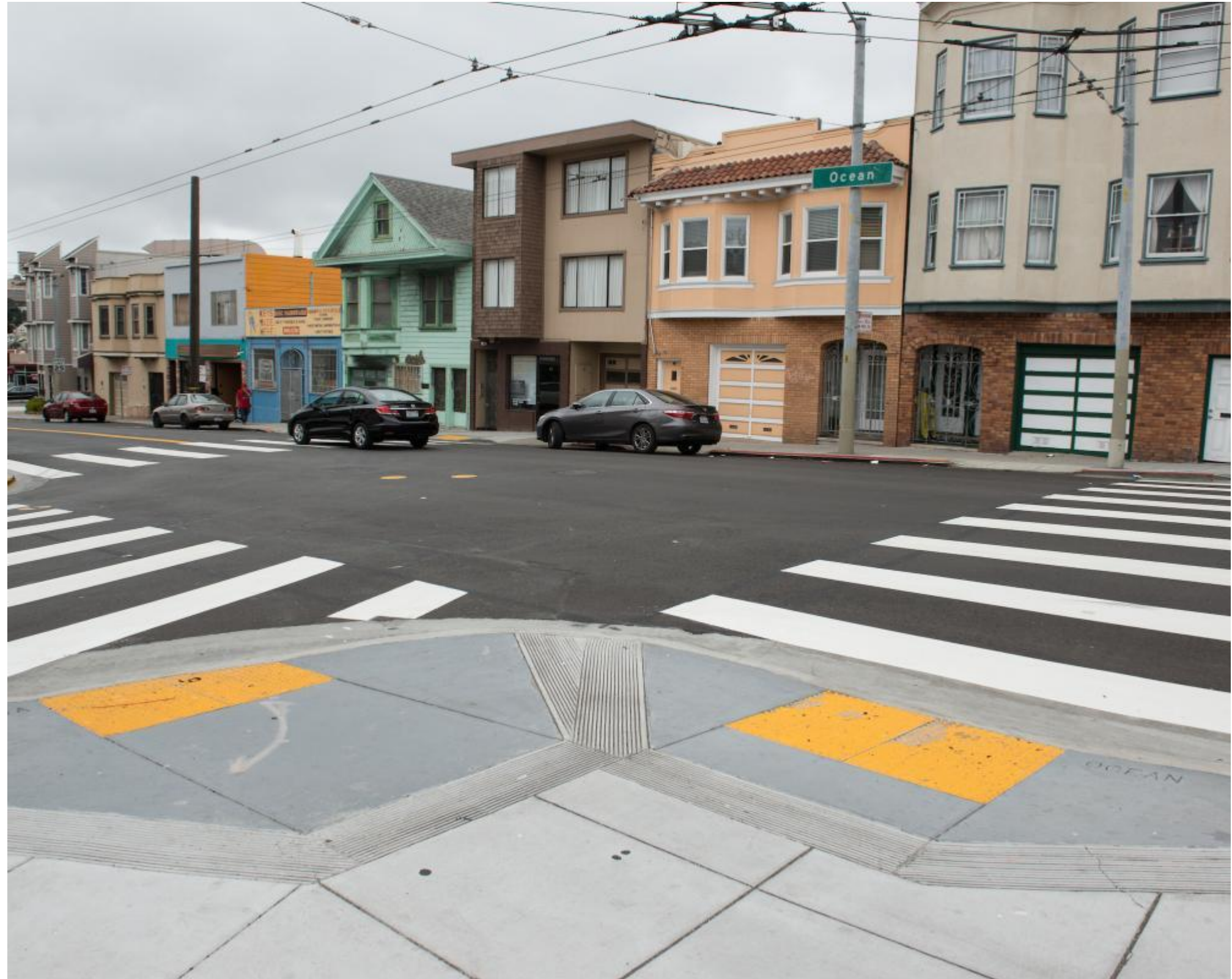
Figure 56. High visibility crosswalk, San Francisco Source: San Francisco Metropolitan Transportation Authority (n.d.)
