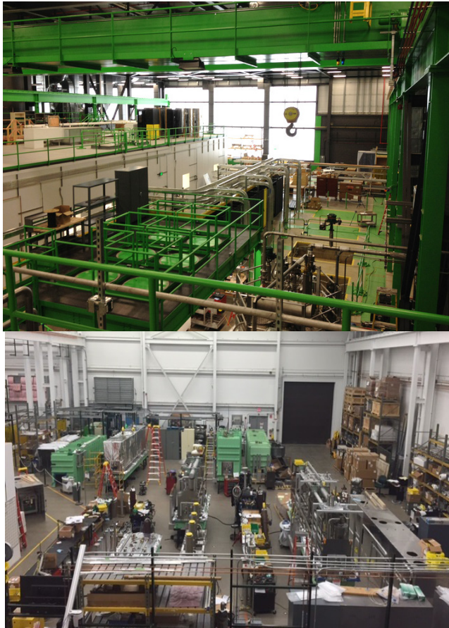
Fig. 13. The SRF highbay (top) and the cryomodule assembly area (bottom) housing six parallel assembly lines delivering more than one cryomodule per month.
