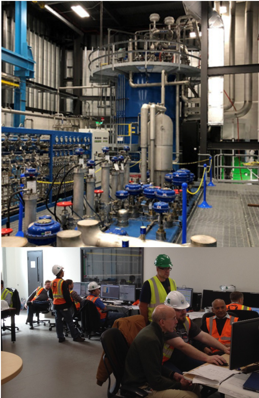
Fig. 4. Commissioning of the FRIB helium refrigeration system (cryoplant) at 4 K in 2017. (Top) The FRIB cryoplant established to supply liquid helium to the entire FRIB accelerator facility. (Bottom) The FRIB cryogenics team during the cryoplant 4 K commissioning in the FRIB cryogenic control room.
