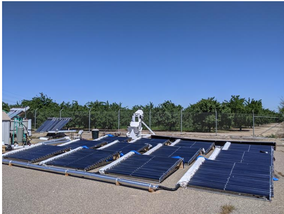
Figure 49: 12 kW ICPC array with insulation and weatherproofing
