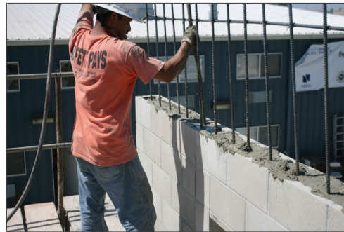
RM wall grouting and consolidation
