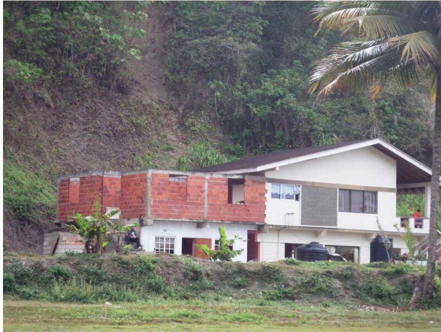
Figure 25. House below steep exposed hillside
