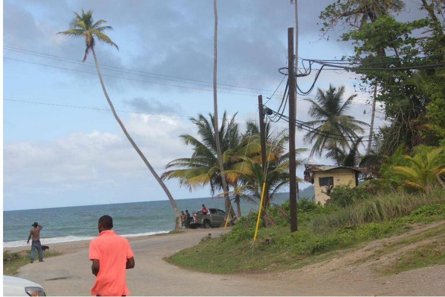
Figure 15. Portion of road in Big Bay-Sans Souci that is frequently flooded by high surges
