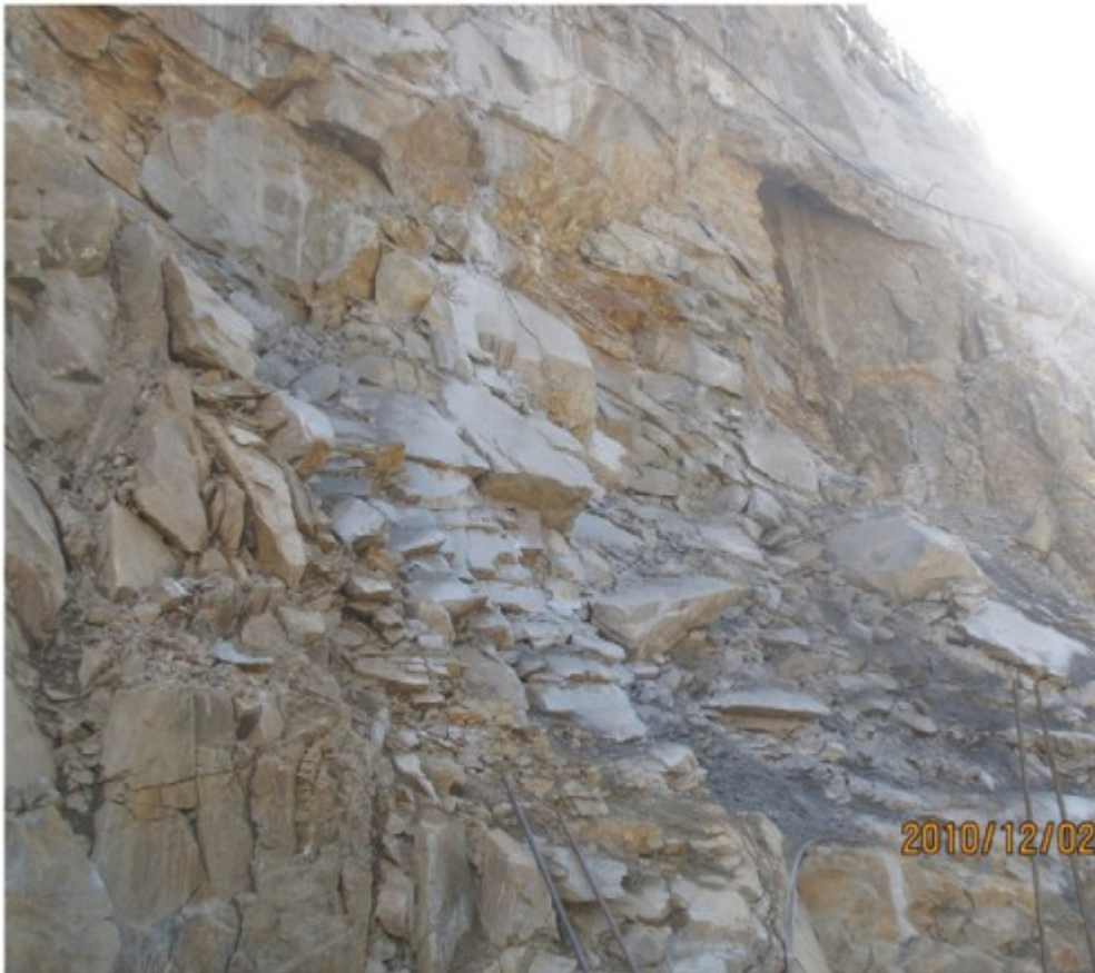
Fig. 6. The fractured and highly permeable rock mass.
