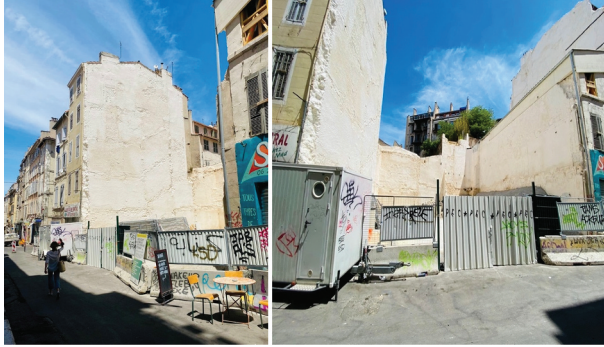
Figure 2. 63–65 Rue d'Aubagne: vacant site of the collapsed buildings, cordoned from public access. © Amir Aziz. June 2021.
