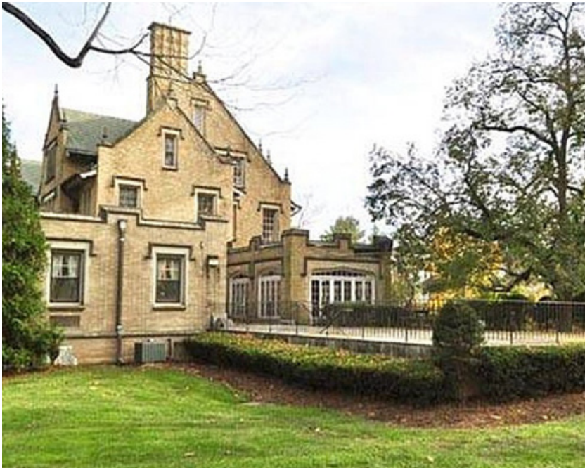
Figure 2 The mansion was retrofitted as a chapel with a “Swamp Yankee” mindset.
