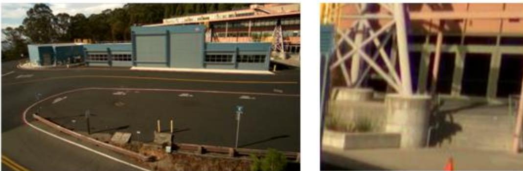
Figure C-8: Images captured from FLEXLAB cameras near LBNL Building 90
