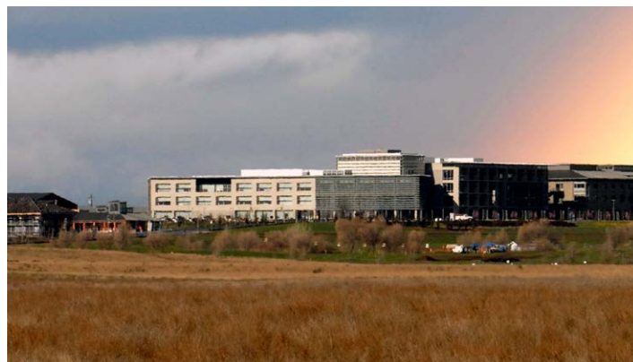
A rainbow touches down over the UC Merced campus. The Central Plant can be seen on the far right; the Science & Engineering building is directly to the left of the plant.
