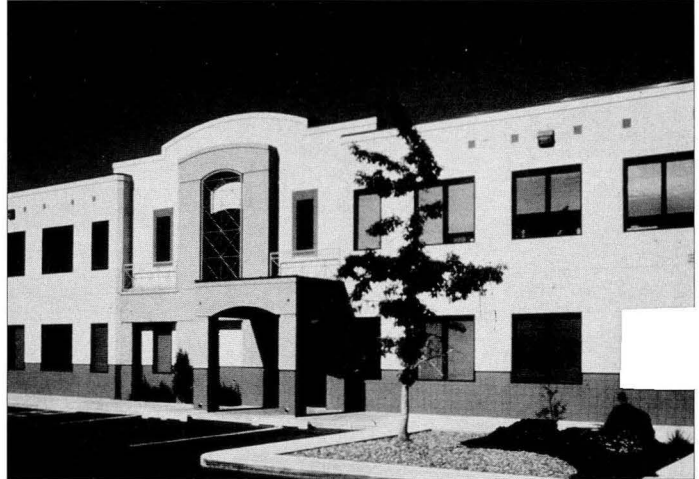
The 13,400 (1,240 m 2 ) square foot Landmark building in Yakima, Washington, one of 28 participating Energy Edge buildings.
