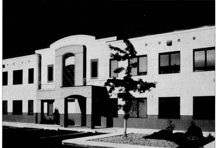
The 13,400 (1,240 m 2 ) square foot Landmark building in Yakima, Washington, one of 28 participating Energy Edge buildings.
