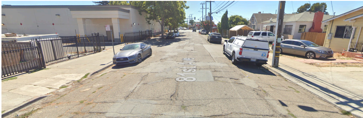
A Google Street View of a segment of 81st Avenue that is included in Calm East Oakland Streets . The project will repave the street, which today is severely rutted, potholed, and patched.
