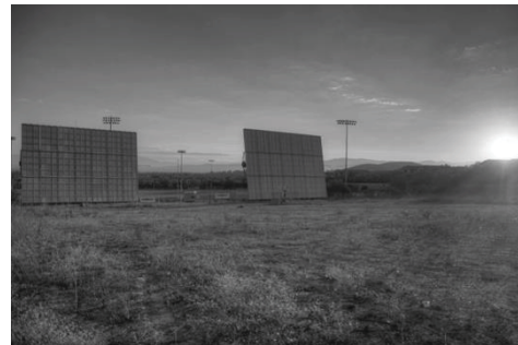
FIGURE 1. Two Amonix CPV-7700 systems installed at the University of California, Irvine.
