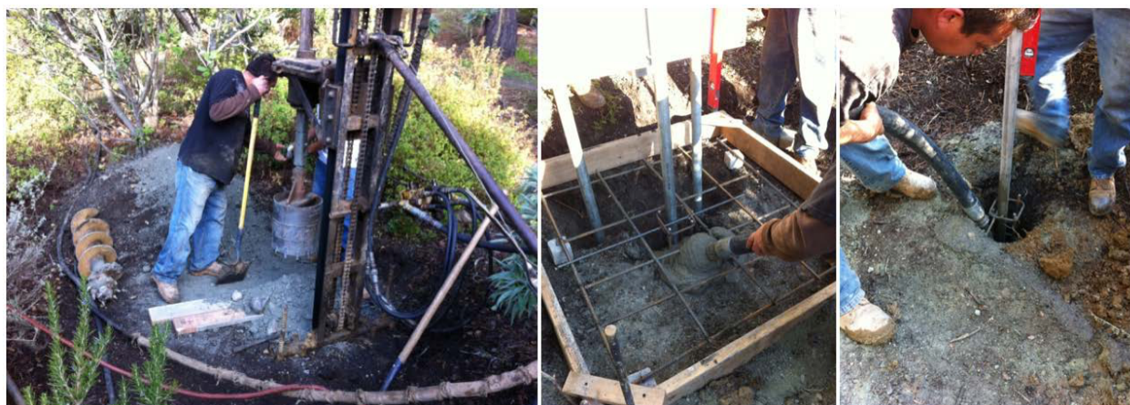
Figure 5-4. cGPS station construction sequence at LRA6 showing (left to right) drilling and excavation, reinforced concrete foundation installation for ancillary monument and reinforced concrete foundation installation for antenna monument.
