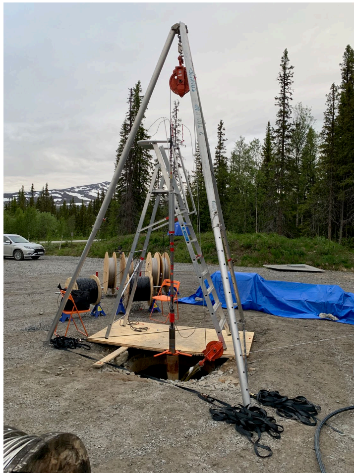
The system with all of the steel tubing connected – only a few more steps before lowering the tool into the borehole!
