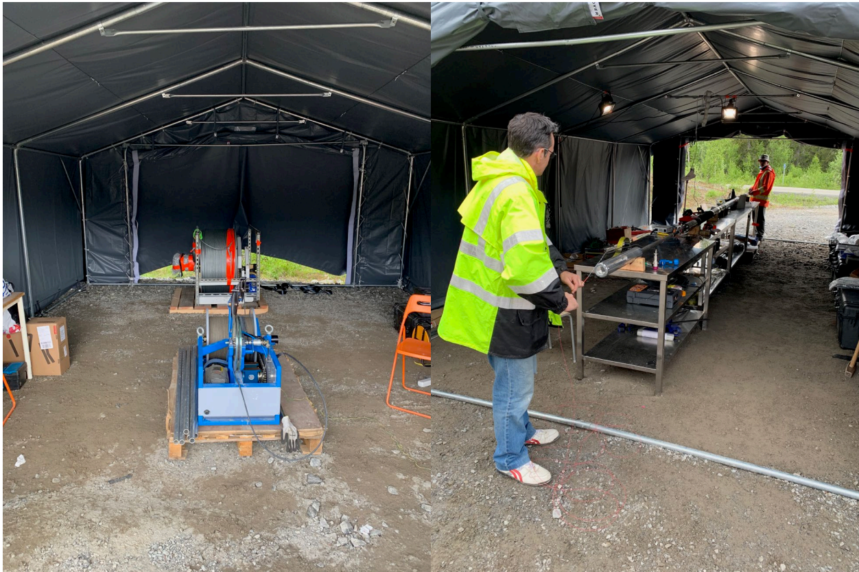
(Left) LBNL winch moved into position with the forklift (Right) Paul and Yves successfully threading wiring through the SIMFIP conduit for the Uppsala gamma tool.
