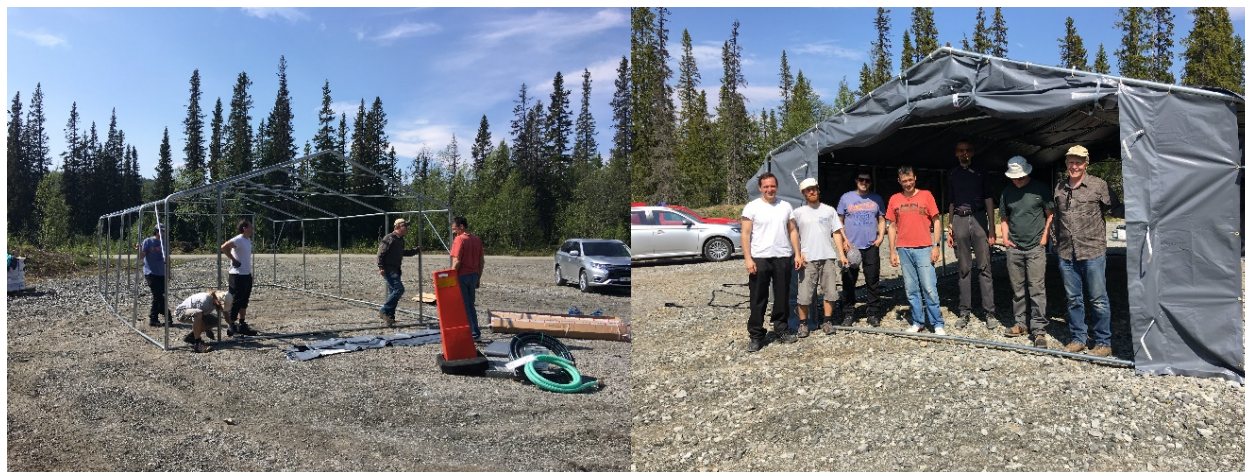
Assembly of tents for building the SIMFIP and hosting the winches.
