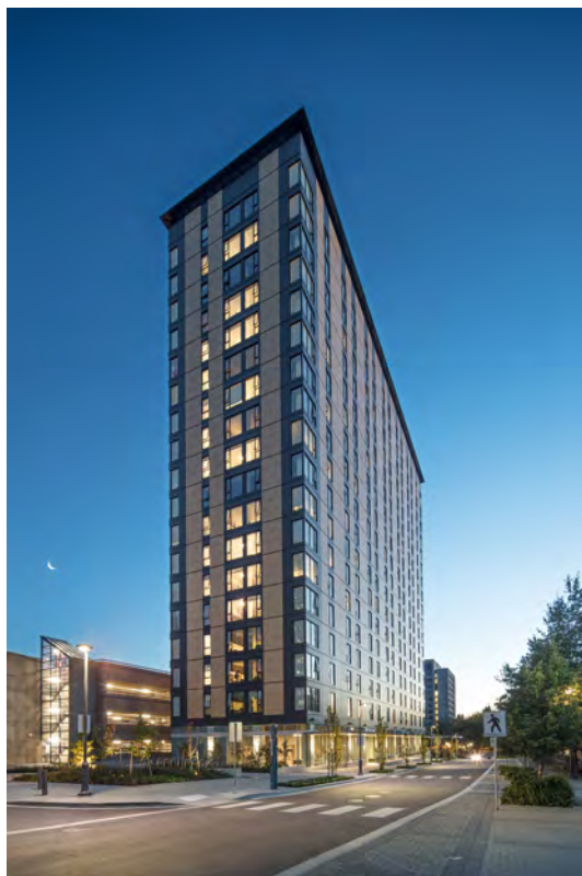
Fig. 14. Brock Commons, an 18-story student residence building at the University of British Columbia, was the world's tallest wooden skyscraper when completed in May 2017. Image CC BY-NC 2.0 University of British Columbia.
