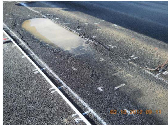
(b) A closer look at the test section
