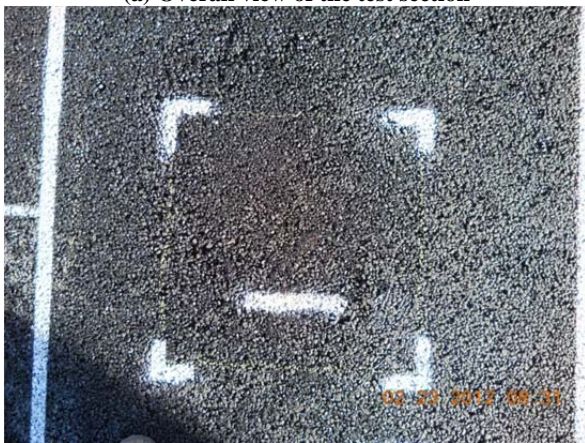
(c) Picture at Station 10 before HVS Trafficking
