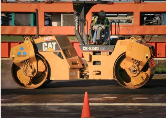
(a) Construction of OGFC
