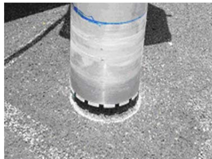
(k) Removal of cores for post-test scanning
