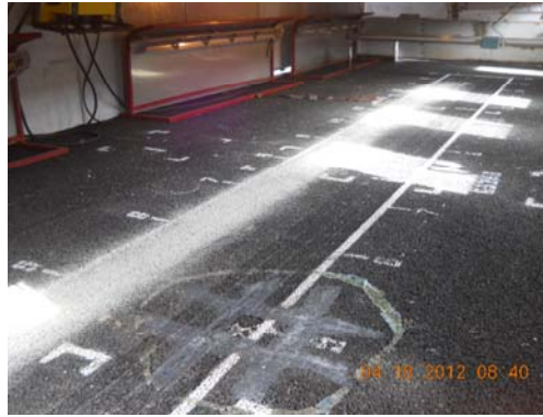
(b) Test section with dust spread on the down-slope wheelpath
