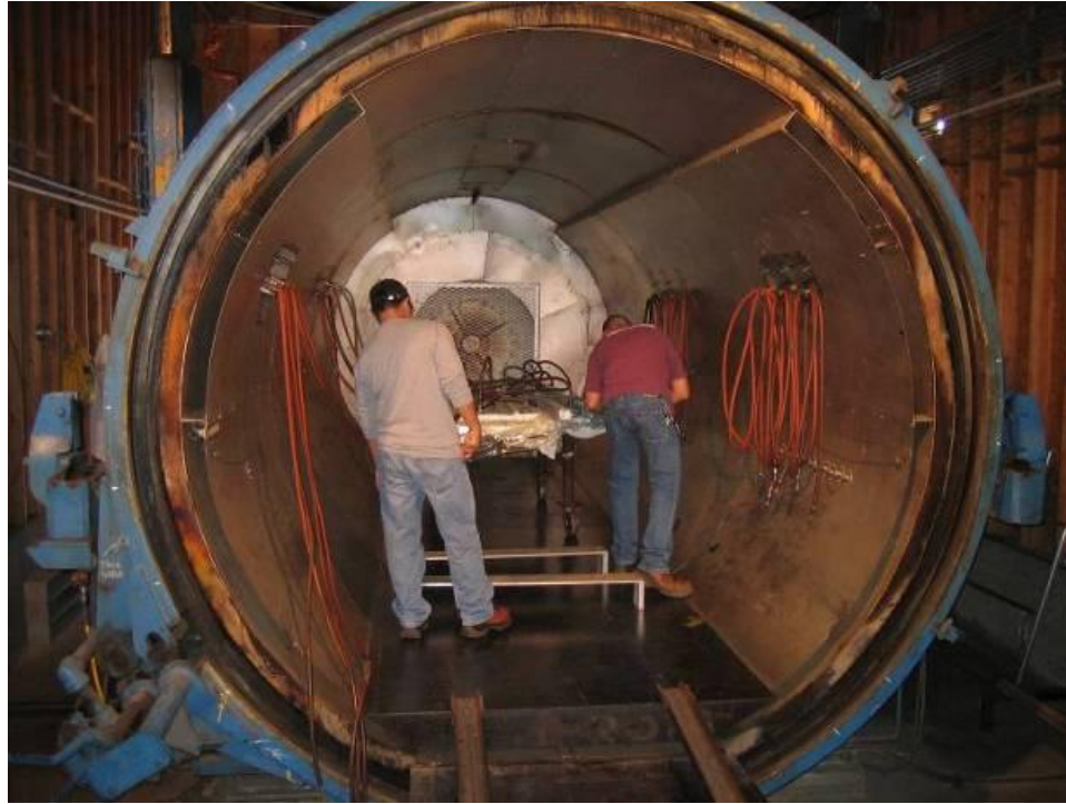
Figure 7-31: Wing components being prepared for cure in an autoclave at Pratt & Whitney Composites.
