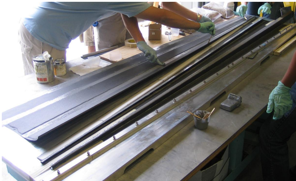
Figure 7-34: Application of structural adhesive onto wing component bondlines.
