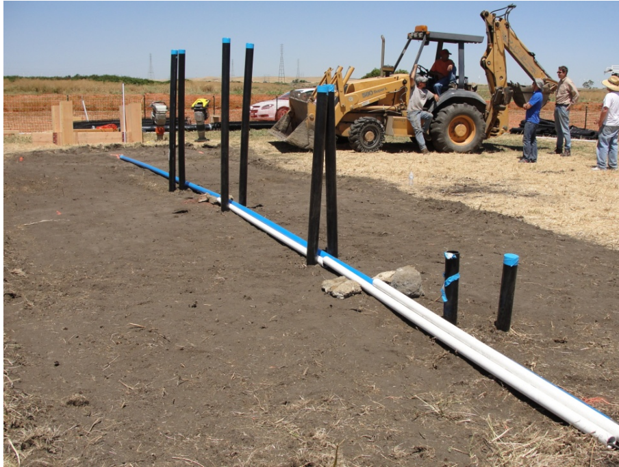
Figure 4.14: In-place inclinometer casing (blue) and PVC guide pipes (white) installed just prior to construction.
