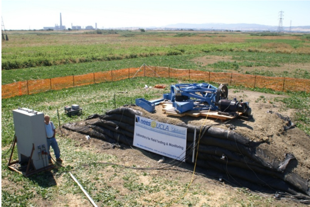
Figure 4.19: Constructed model embankment with NEES@UCLA MK-15 shaker.
