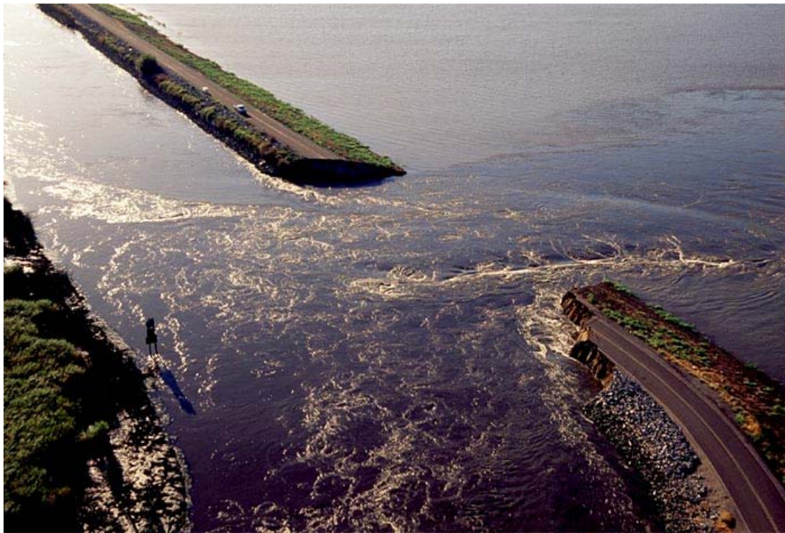
Figure 1.4: Aerial photo of the 2004 Jones Tract failure. (Lund et al. 2007)
