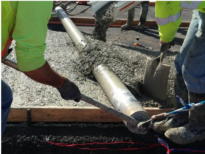
Concrete Paving of the Full-Scale Sections. A hand-operated roller screed was used for placement and consolidation of the concrete. This tool was selected because of the relatively small configurations of the concrete placements and the high workability of the mixes. Minimal additional vibration was required.
