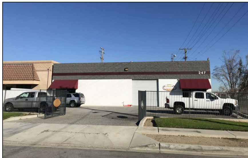
Figure 7. Photo of the outside of the selected warehouse facility for manufacturing.
