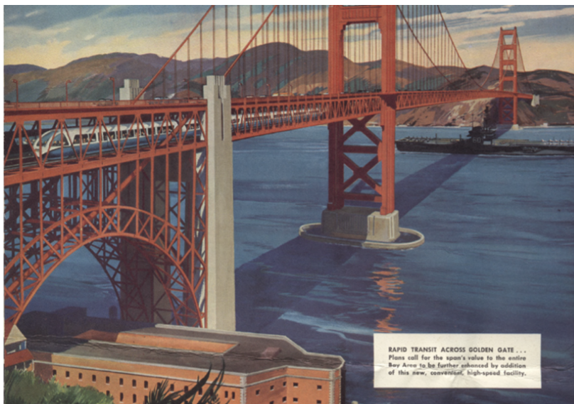
Figure 1.7: Rendering of rapid transit trains on a proposed second deck of the Golden Gate Bridge. America Moves Ahead with Rapid Transit, General Electric, 1961.
