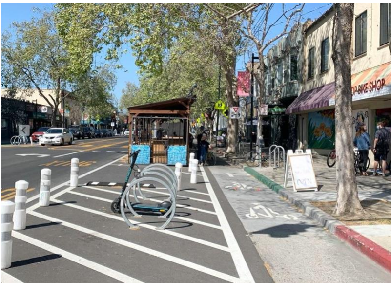
Figure 11. Short segment of protected Class 4 cycle track on Telegraph Ave. Oakland, CA
