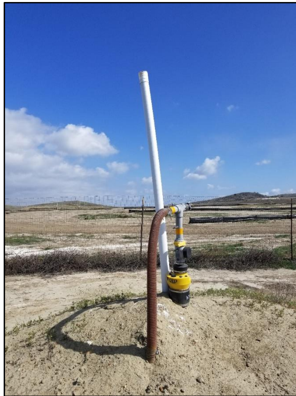
Figure 1.4 Exposed landfill gas collection pump infrastructure at Prima Deshecha landfill. Photo taken by Brenna Biggs during April 2018.
