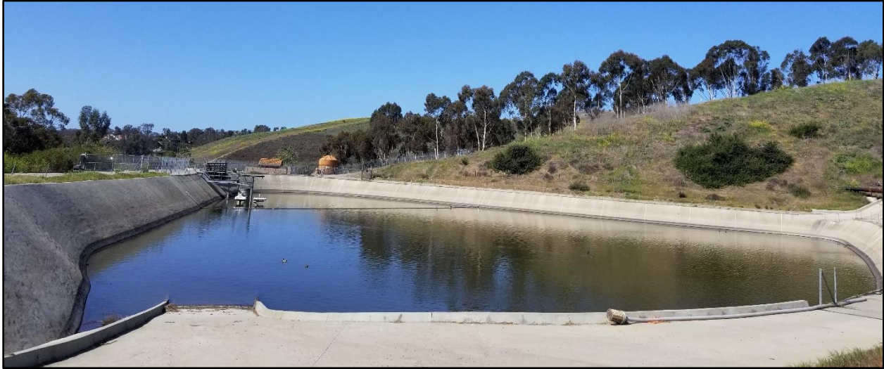
Figure 1.5 Filled water runoff and desilting basin at Prima Deshecha landfill in Orange County. Photo by Brenna Biggs in April 2018.
