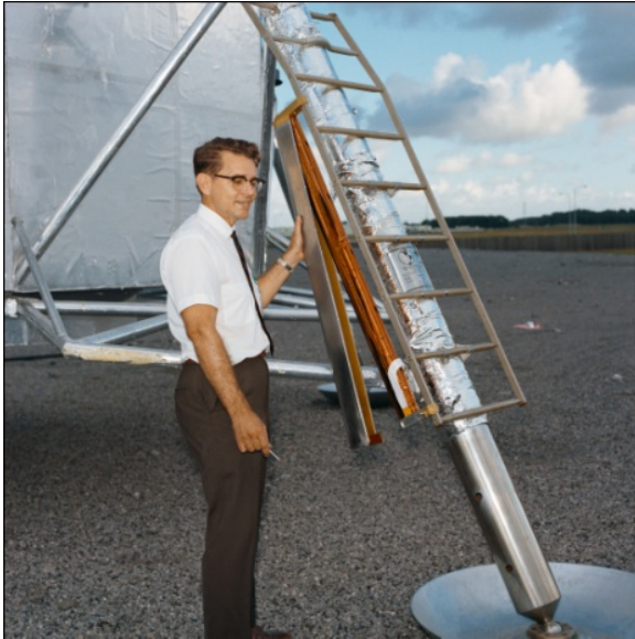
Figures 24–25: A NASA engineer (on Earth) indicates the location where the lunar flag assembly was mounted on the ladder of the lunar module for Apollo 11 and 12. After removing the protective shroud (left), he removes the Velcro strips in order to open the insulation package (right). (NASA JSC Photos S69-38755, S69-38756).
