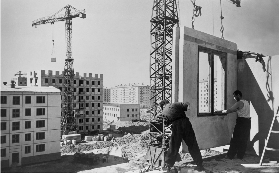
Fig. 3.4 Construction workers of the Kulikov building brigade set a pre-fabricated concrete wall section in place on the fifth floor of a new Moscow apartment block, June 1960. Everett Collection / Alamy EG6PT5.
