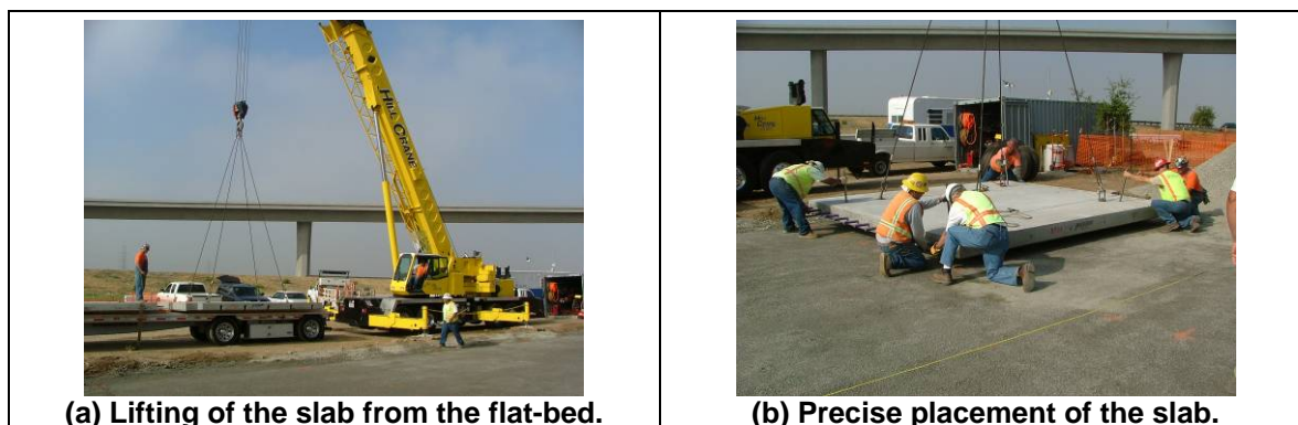
Figure 7. Placement of the pre-cast slabs.
