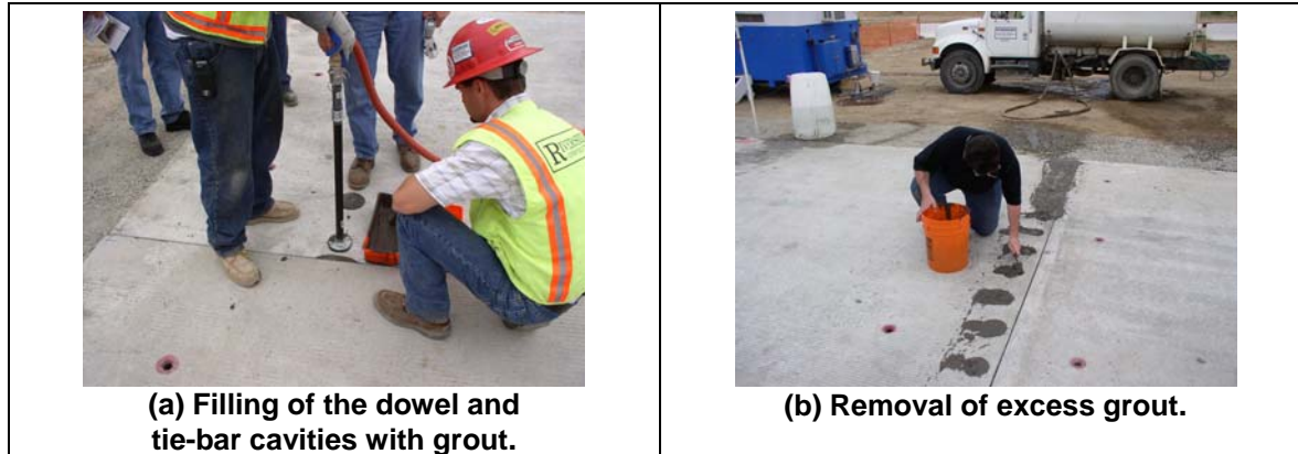
Figure 13. The grouting of the dowel and tie-bar cavities.
