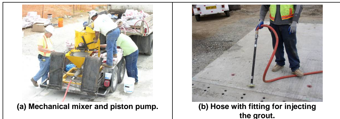
Figure 12. Basic components of the grouting equipment.
