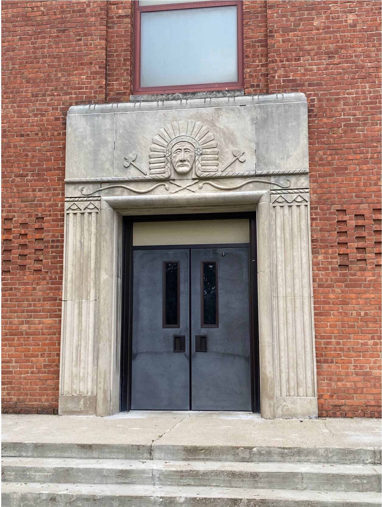
Figure 6. An entryway, Indian Springs Elementary, Columbus, Ohio.
