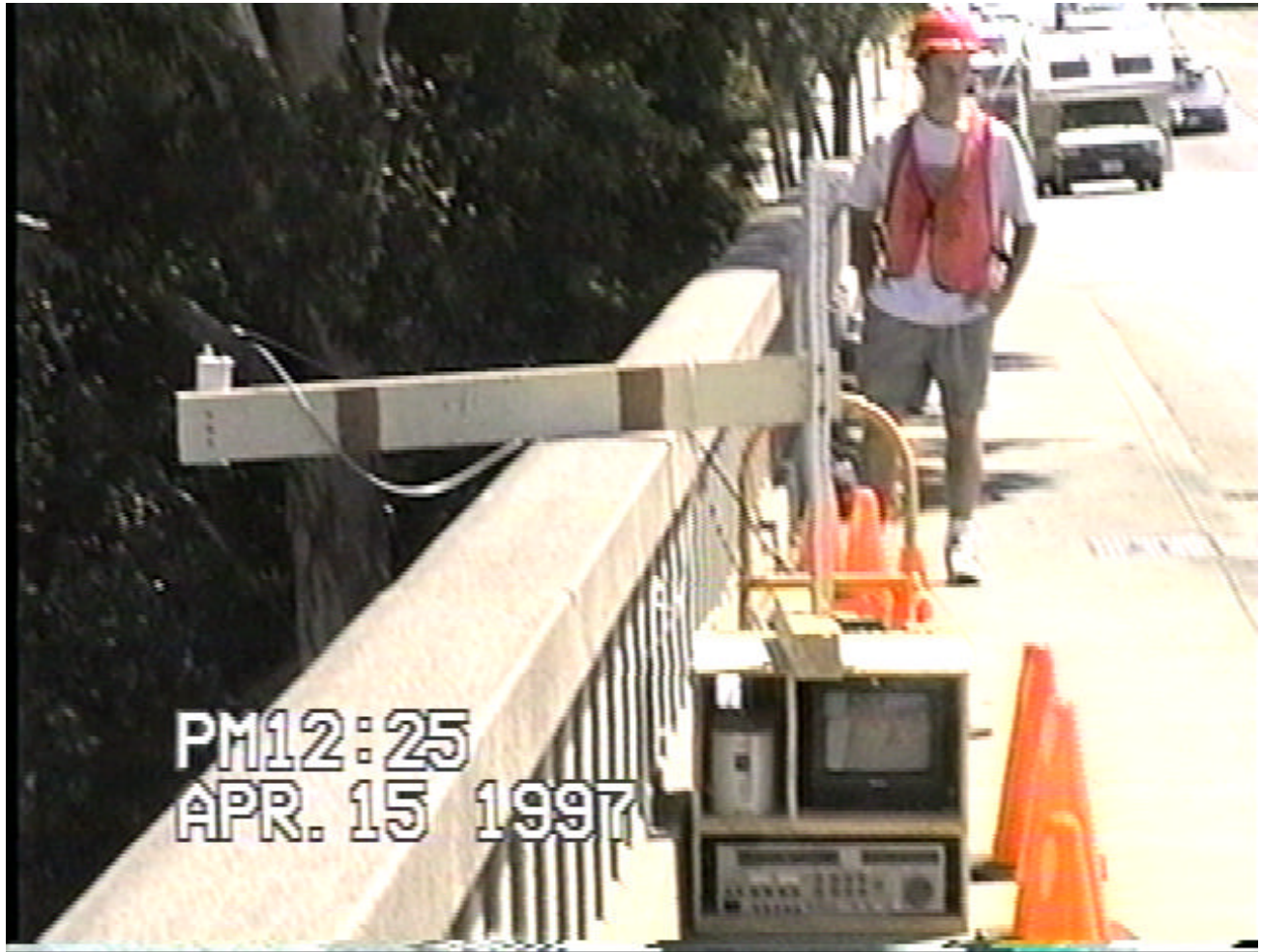
Figure 6. Typical Daytime Deployment of Data Acquisition System on Freeway Overcrossing.
