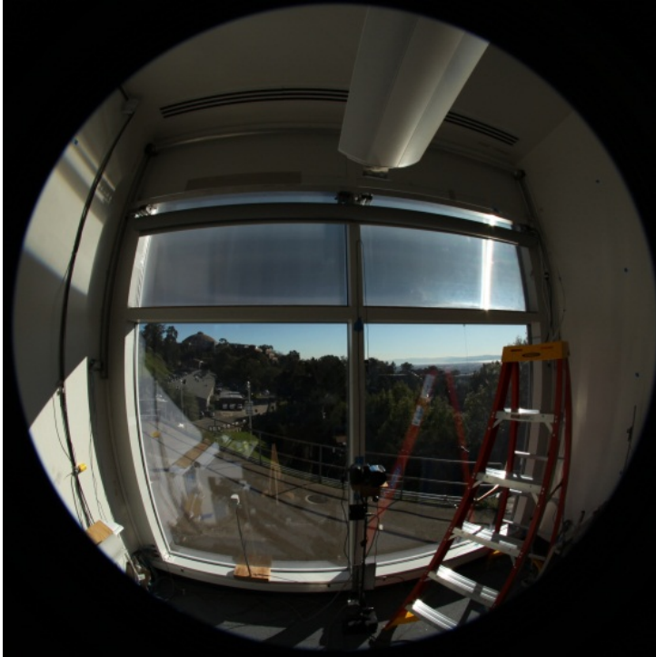
Fig. 7. Interior view of the film installed in the two upper clerestory windows. The bright arc of sunlight being redirected to the viewer is visible close to the right-most edge of the right window.
