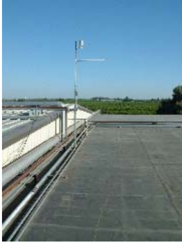
Figure 36. Kaprielian Brothers Packing Company (Cold Storage) Facility in Reedley: Weather tower
