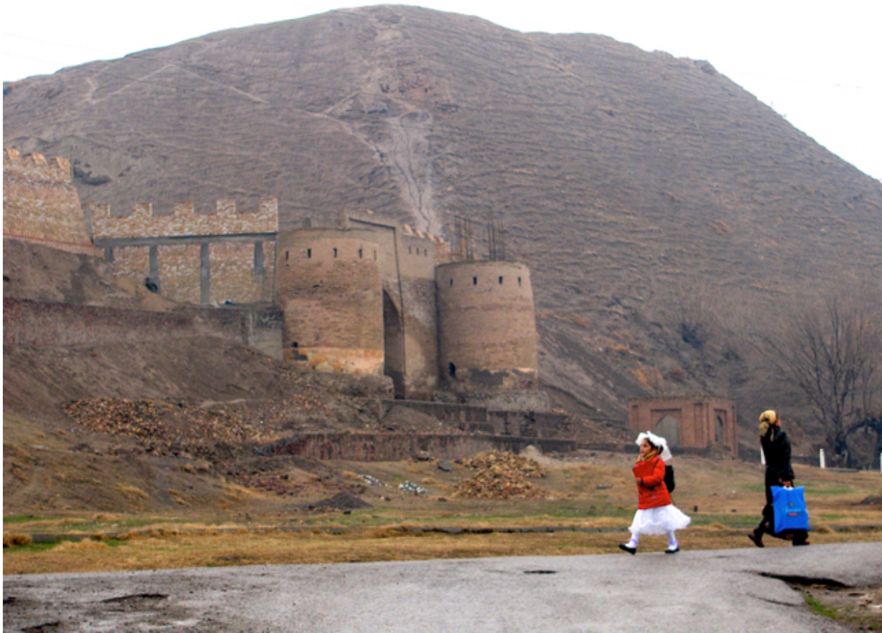
Hissar or fortress located in the suburb of Dushanbe under re-construction in 2011. Copyright Khashayar Beigi
