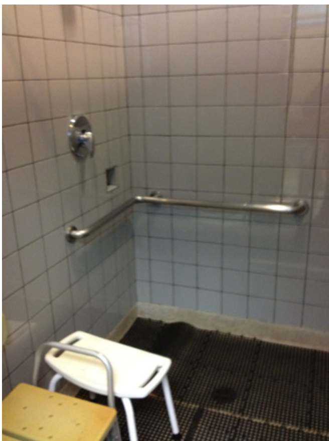
Figure 4. Shower. The shower for washing off the topical medications with mineral oil and soap. Shower is equipped with safety mats to prevent the floor from getting slippery. Safety handles are also present and important, especially for the elderly.
